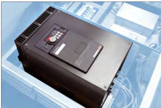
Frequency converter in the Hänel Lean-Lift® EcoDrive®
